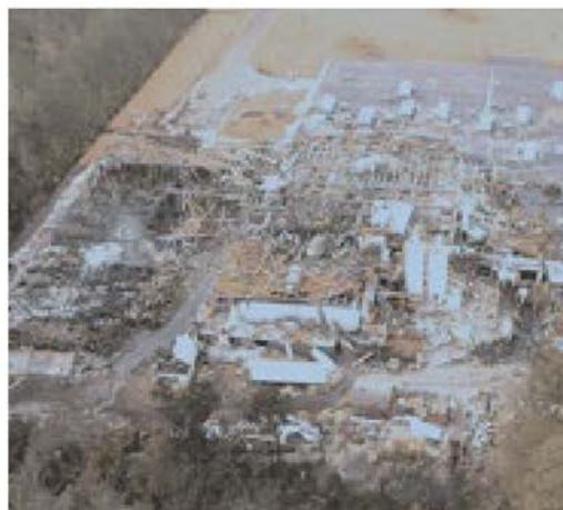
A pharmaceutical plant after a dust explosion.
