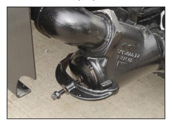
2" Y-strainer at water fill - Assembled
