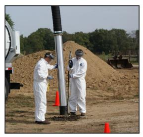
pull air into the pipe to move material. The end is serrated with small holes; if the end is submerged no air is pulled in through the holes. Symbols Operation
