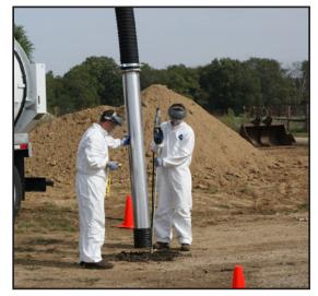
pull air into the pipe to move material. The end is serrated with small holes; if the end is submerged no air is pulled in through the holes.
