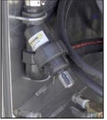
Y-strainer shown assembled and with element removed for cleaning.
