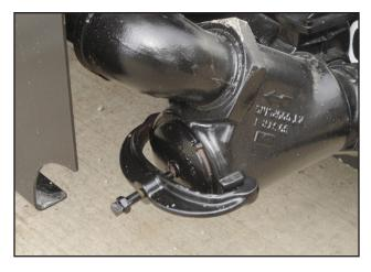
2" Y-strainer at water fill - Assembled
