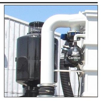
The pressurized air is used to clean the baghouse at certain intervals during the operation. The length of the cycle is controlled at the master control panel. The air cannon will fire approximately every 60 seconds.
