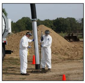
pull air into the pipe to move material. The end is serrated with small holes; if the end is submerged no air is pulled in through the holes.
