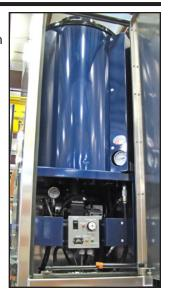
The controls are located under the water heater inside the cabinet on all versions. The 400,000 and 800,000 BTU units use the same control panel.
