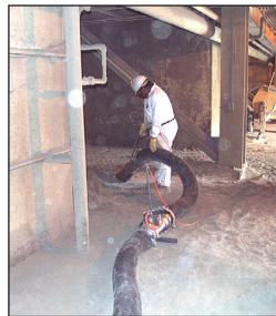
Shown is an example of a good vacuum hose run. The hose is the same size from the truck to the hose end. The Safety tee is located for good operator access and a hose end is being used.
